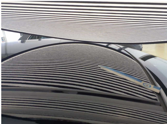
Damage 2: Roof: Roof - dent(s) - Smooth repair work
