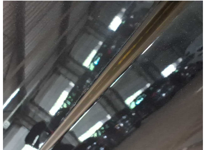
Damage 5: Sliding door, right: Sliding door with glass panel (Einschlüsse, matt poliert, wellig, kante unsauber) - Unprofessionally repaired - Repair and paint
