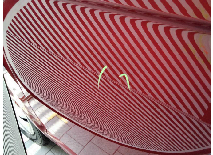
Damage 7: Sliding door, right: Sliding door with glass panel - Dent / paintcoat damage - Paint
