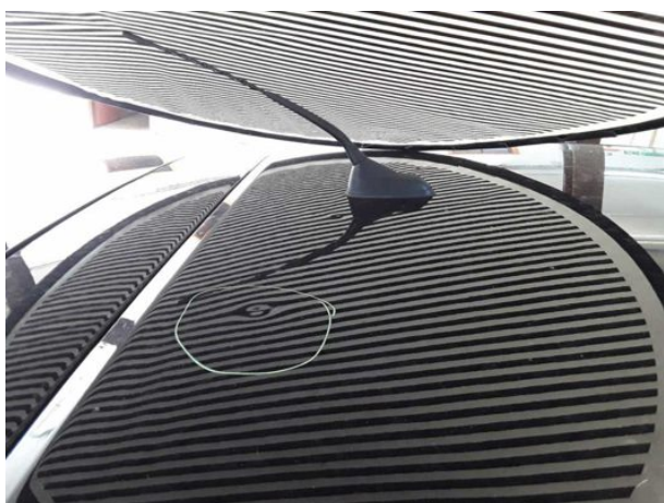
Damage #10: Roof: Roof - dent(s) - Smooth repair work
