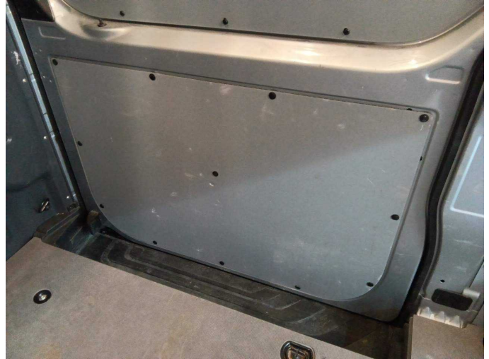
Damage 7: Sliding door, right: Trim (Unten) - Holes - Replace
