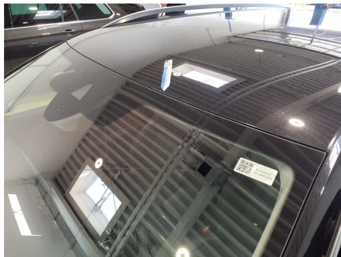
Damage 10: Roof: Roof - Corrosion - Repair and paint
