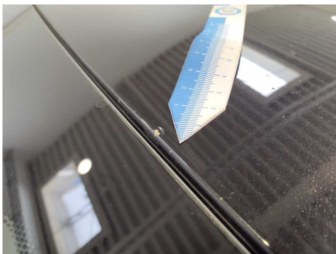
Damage 10: Roof: Roof - Corrosion - Repair and paint
