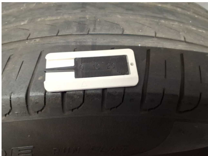
Damage 9: 2nd wheel set: 2 tyres - Worn - Replace
