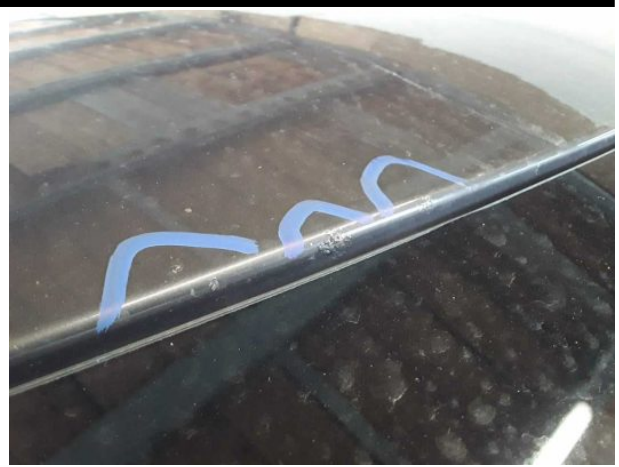
Damage #10: Roof: Roof - Corrosion - Repair and paint
