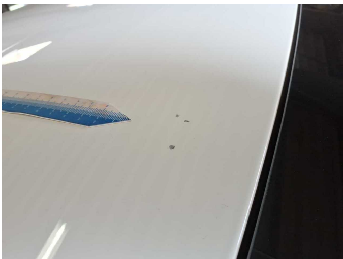
Damage 15: Roof: Roof - Stone chips - Paint
