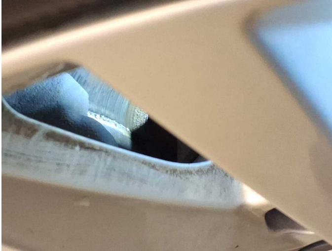
Damage 10: Braking system: Brake discs and brake pads - front (Tragbild mangelhaft) - Worn - Replace
