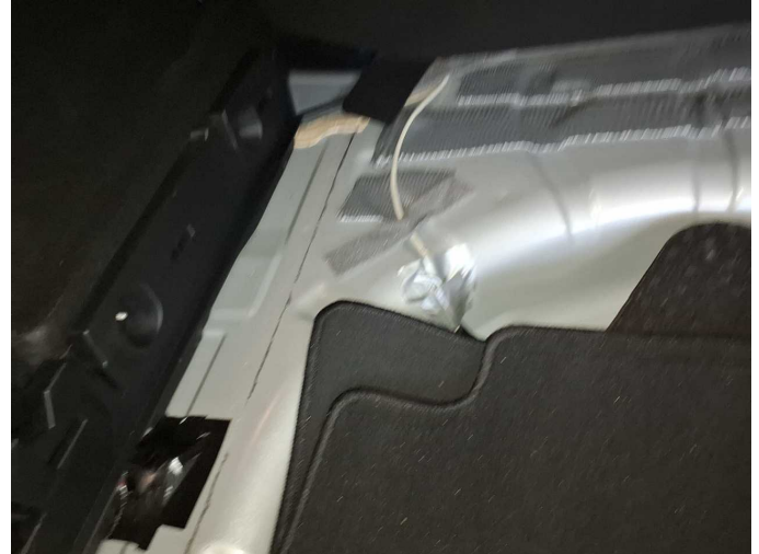
Damage 1: Electrical system: Cable strand (Kabelführung von Frontbereich in Laderaum) - Differs from the original configuration - Un-/install
