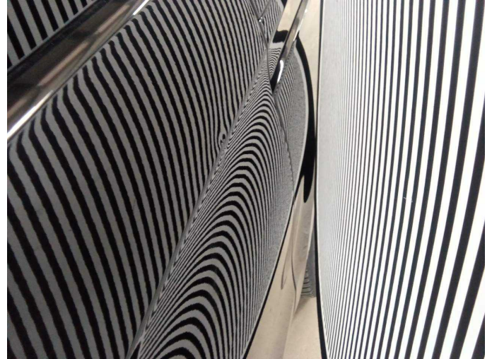
Damage 6: Sliding door - left side: Sliding door - Dent / paintcoat damage - Repair and paint
