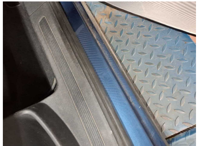
Damage 9: Side panel - rear right side: Sill - dent(s) - Smart repair
