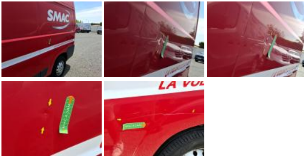
Shutter / cover F, Missing, Replace
