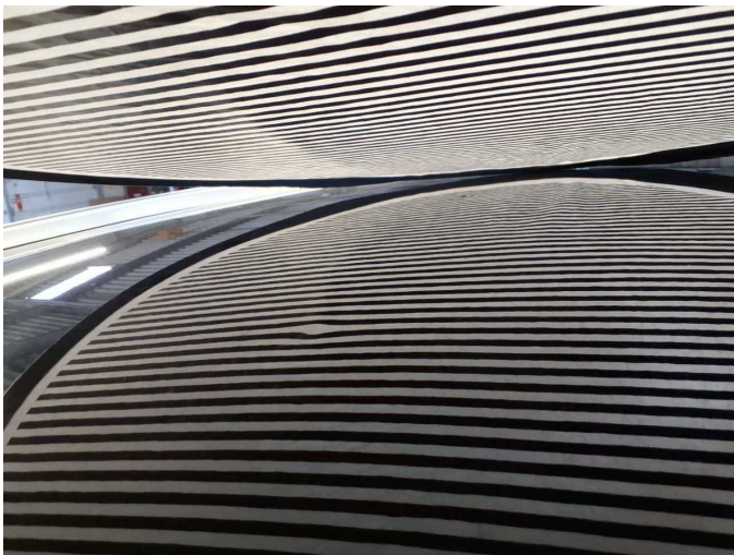
Damage 16: Roof: Roof - dent(s) - Smooth repair work
