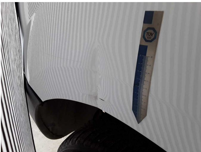
Damage 7: Side panel - rear right side: Side panel (Unterhalb) - Deformed - Repair and paint
