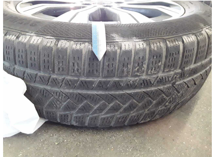
Damage 1: 2nd wheel set: 2 tyres - Worn - Replace
