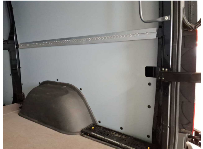
Damage 1: Trim / covers: Cargo area - lining - right side (unten) - Damaged - Loss in value
