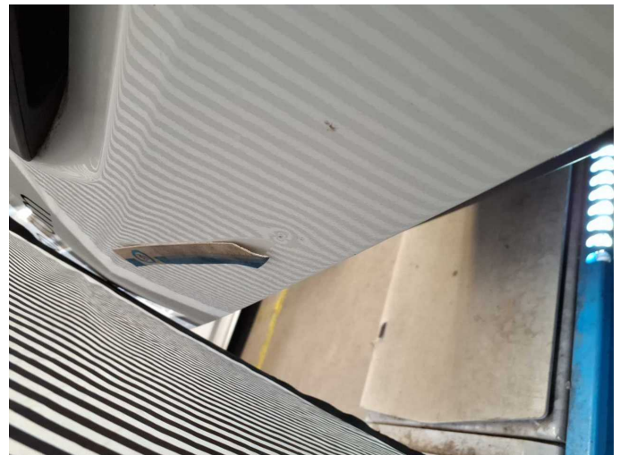
Damage 6: Boot lid / rear door: Boot lid - Dent / paintcoat damage - Smart repair
