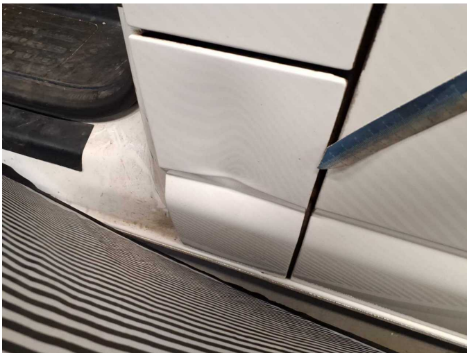
Damage 10: Side panel - rear left side: Side panel (Blende unter'm Tank) - Deformed - Replace
