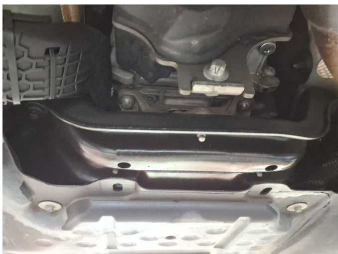
Damage 1: Body: Underbody (Verölt) - Leaking - Perform diagnosis
