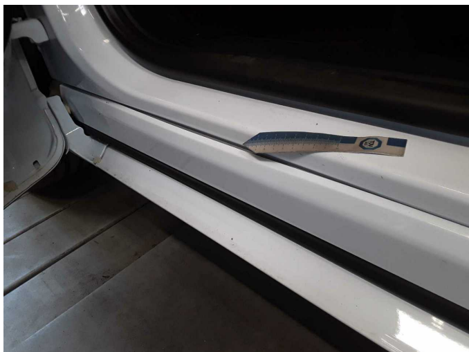
Damage 6: Sill - left side: Trim - Damaged - Replace
