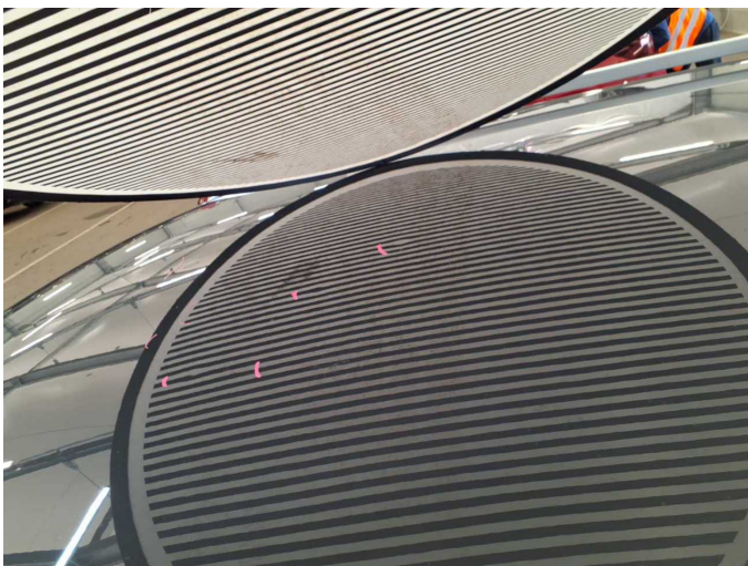
Damage 7: Body: Body - Damage by hail - Smooth repair work
