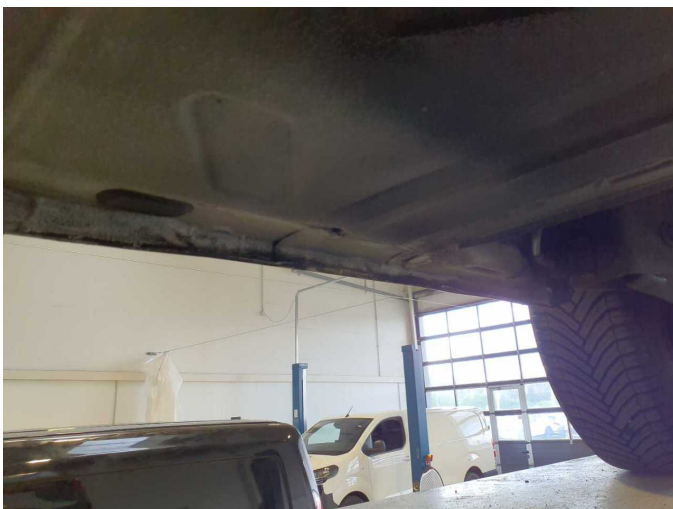
Damage 5: Sill - right side: Sill - dent(s) - Smart repair
