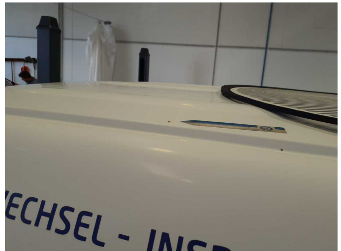
Damage 14: Roof: Roof - Corrosion - Repair and paint
