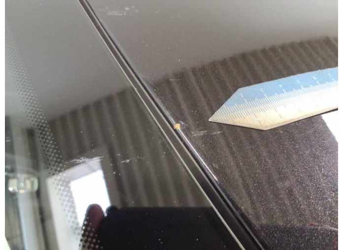
Damage 10: Roof: Roof - Corrosion - Repair and paint
