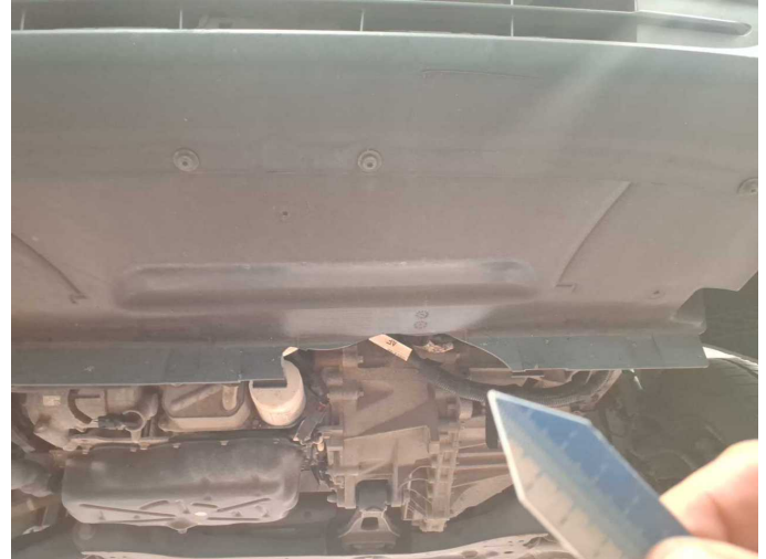
Damage 3: Engine: Engine cowling lower front - Broken / torn - Replace
