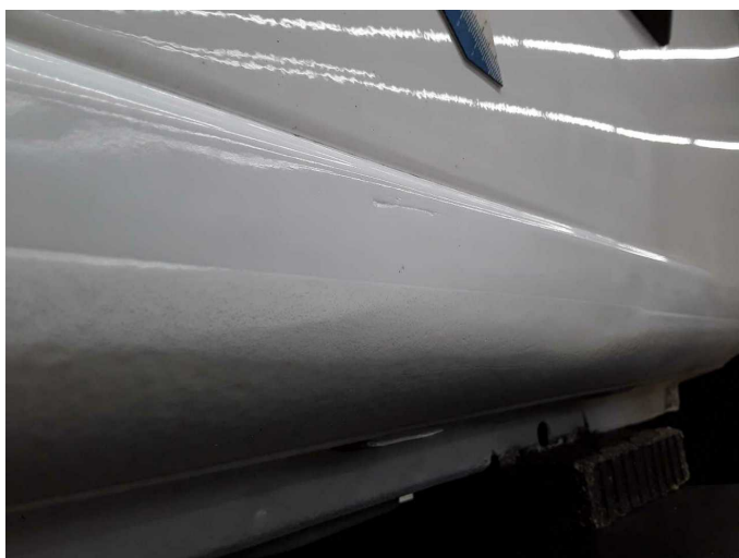
Damage 13: Sill - left side: Sill - Unprofessionally repaired - Repair and paint
