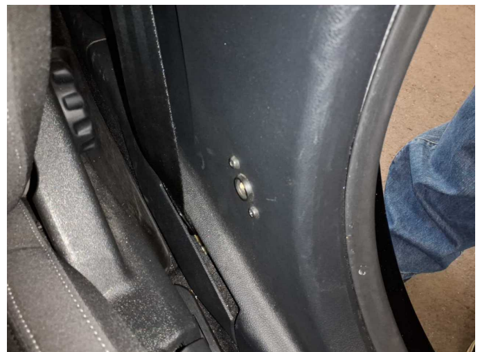
Damage 6: Body: B-pillar - left side (Fehlbohrungen) - Differs from the original configuration - Replace
