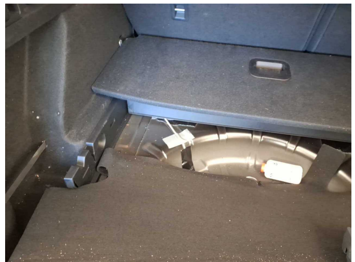
Damage 2: Electrical system: Cable strand (Kabelführung von Frontbereich in Laderaum) - Differs from the original configuration - Un-/install
