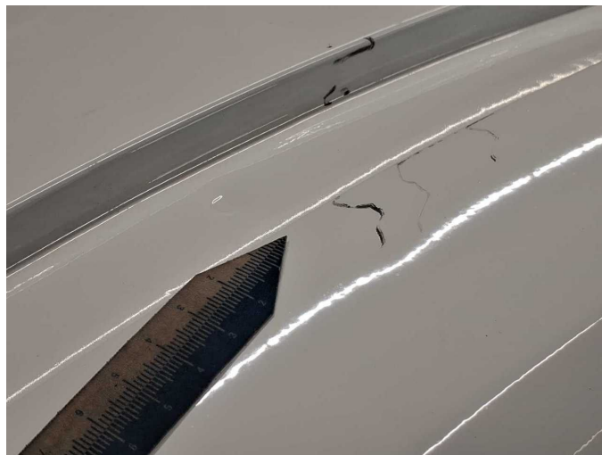
Damage 12: Roof: Roof - Scratch(es) - Paint
