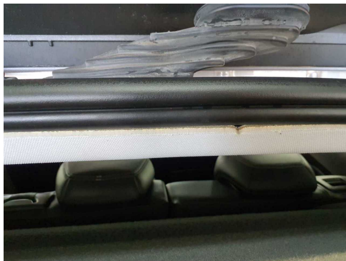
Damage 6: Trim / covers: Roof lining - Loose - Repair
