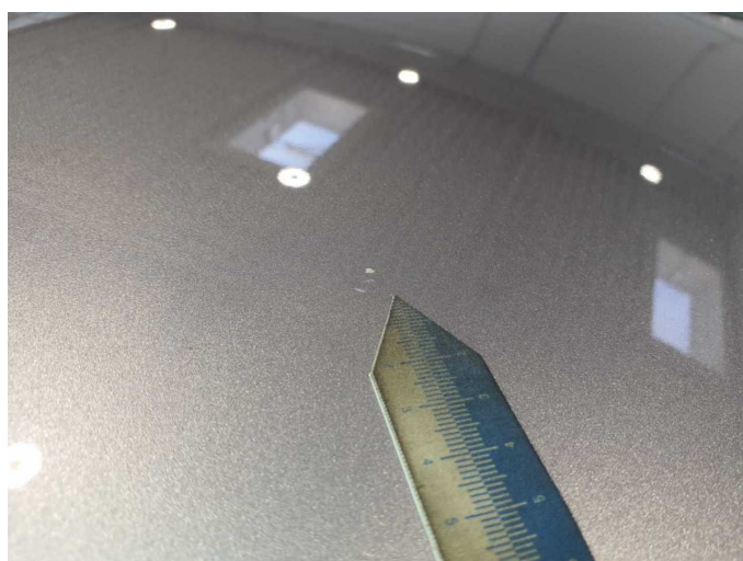
Damage 13: Roof: Roof - Stone chips - Loss in value
