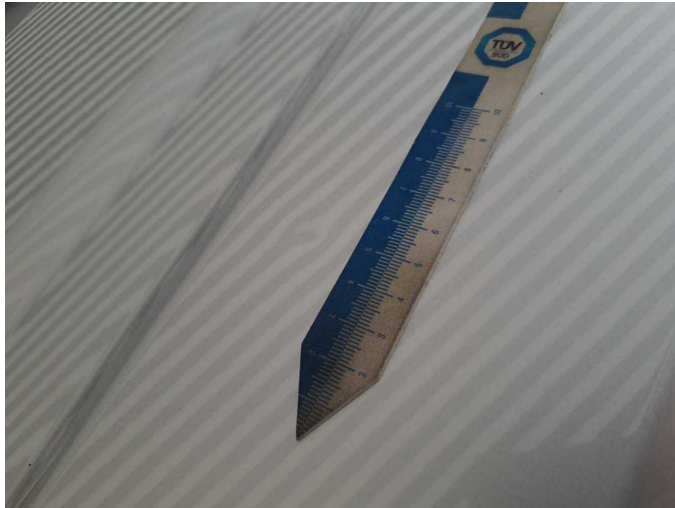
Damage 8: Roof: Roof - Deformed - Repair and paint
