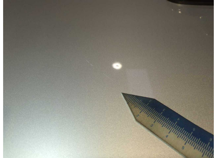
Damage 12: Roof: Roof - Scratch(es) - Paint
