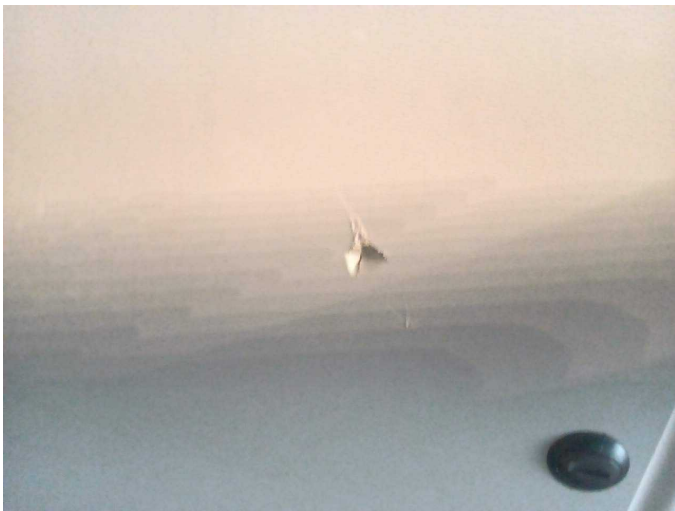
Damage 1: Sliding door, right: Trim - Holes - Replace
