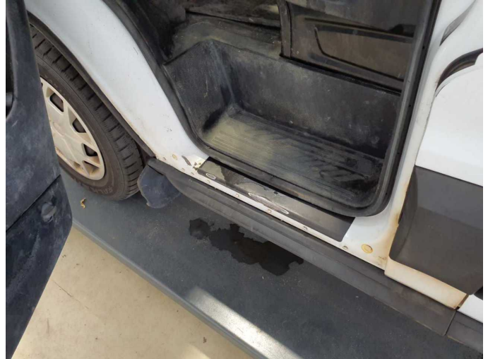
Damage 11: Sill - left side: Sill - Corrosion - Repair and paint
