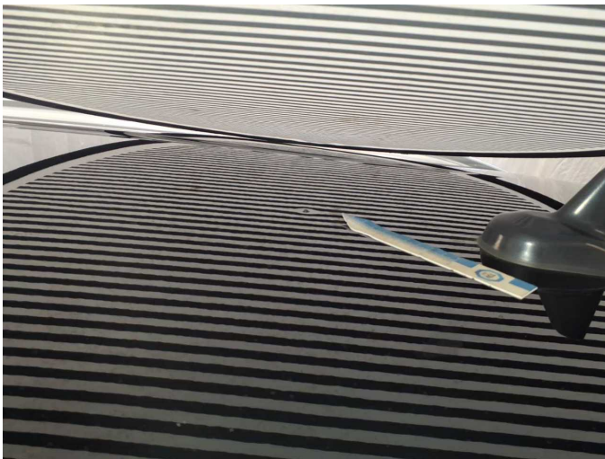
Damage 3: Roof: Roof - dent(s) - Smooth repair work
