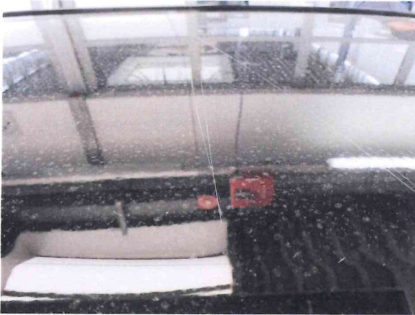
Unfall 1: Dach, Front
