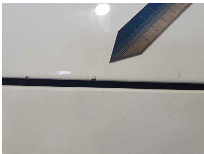
Damage 9: Bonnet: Bonnet - Corrosion - Repair and paint
