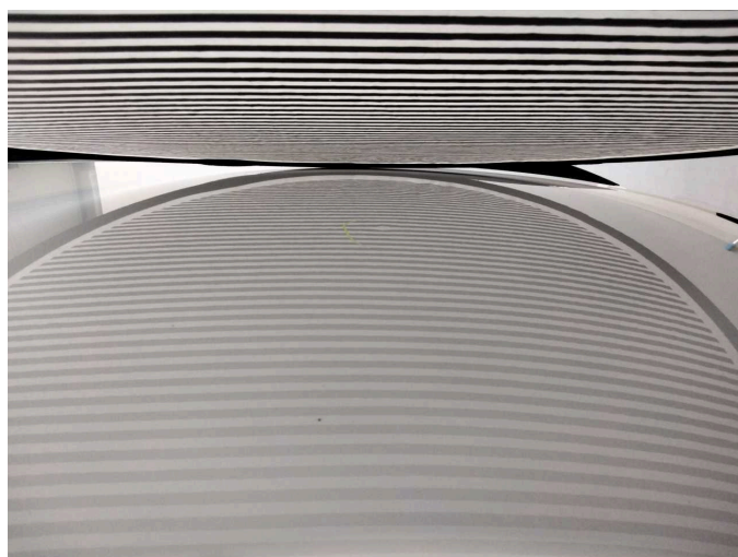
Damage 3: Roof: Roof - dent(s) - Smooth repair work
