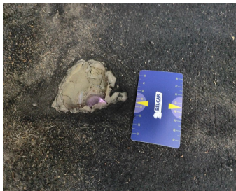
Interior / Floor Covering / Replace-hole
