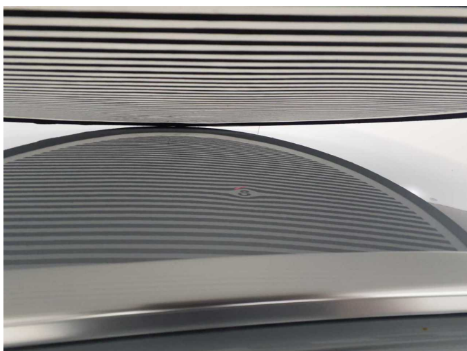
Damage 5: Roof: Roof - dent(s) - Smart repair
