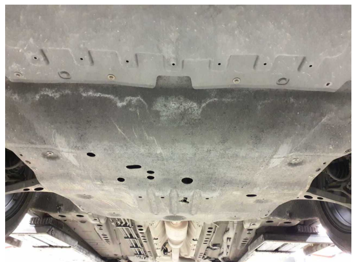
Damage 1: Body: Underbody panelling (VM) - Broken / torn - Replace
