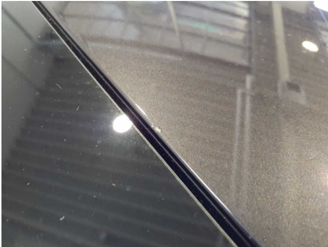
Damage 11: Roof: Roof - Corrosion - Repair and paint
