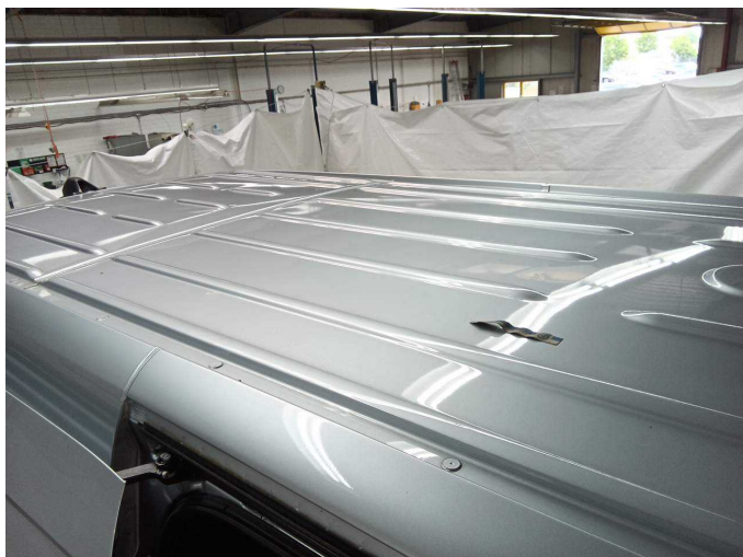
Wear and tear 4: Roof: Roof - dent(s) - No deduction
