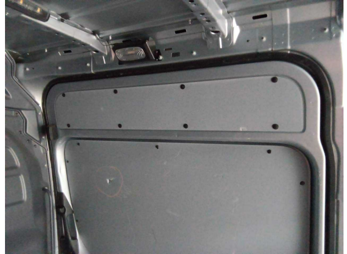
Damage 4: Sliding door, right: Trim - Holes - Replace
