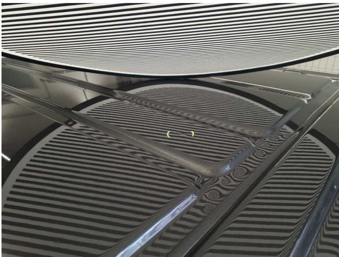
Damage 14: Roof: Roof - Damage by hail - Smooth repair work
