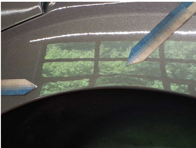
Damage 15: Side panel - rear left side: Side panel (Lack wellig) - Unprofessionally repaired - Repair and paint
