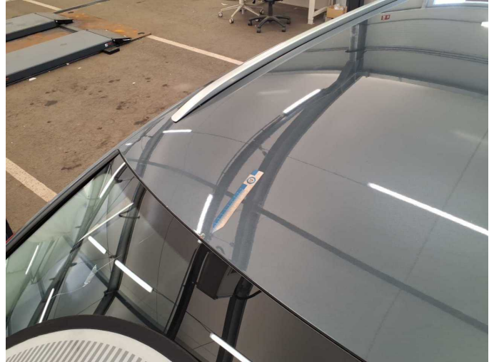
Damage 10: Roof: Roof - Corrosion - Repair and paint
