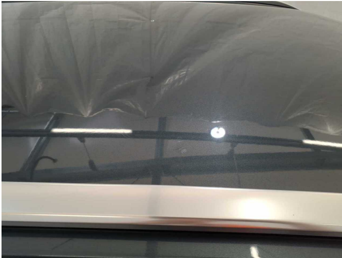
Damage 10: Roof: Roof - Corrosion - Repair and paint
