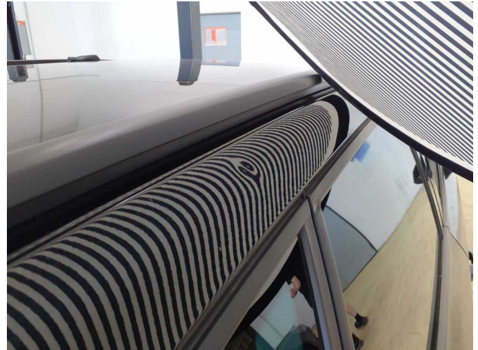
Damage 8: Roof: Roof rail - right side (Einschlüsse) - Unprofessionally repaired - Repair and paint
